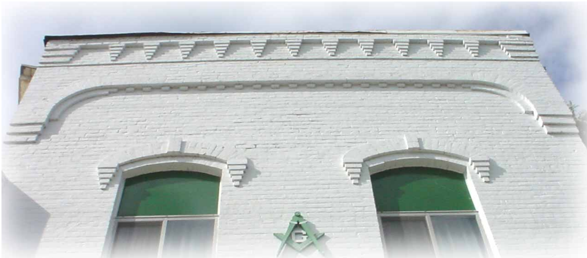
Brickwork on Bank Building-Masonic Building
